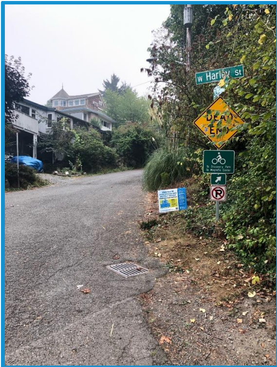
Signage: Project signage on the north approach
